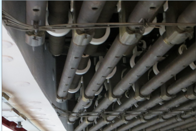
Illustration 1: Angled Air Tubes & Elements
